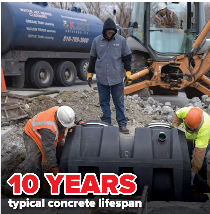
replacement of corroded concrete unit with Schier model GB-250
