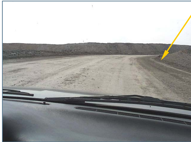
Constant cross fall and drain for water
