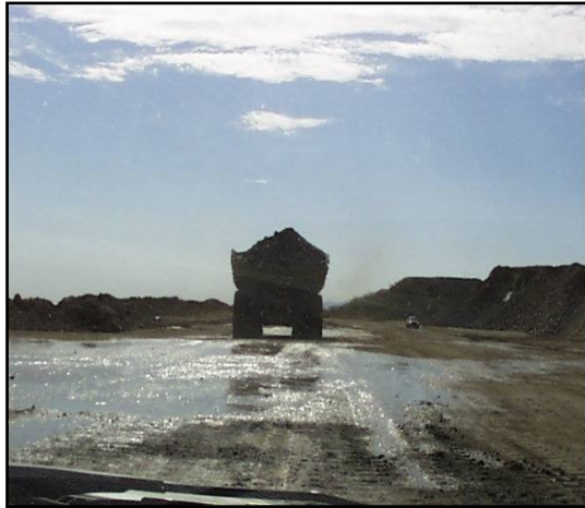
Excess water sprinkling
