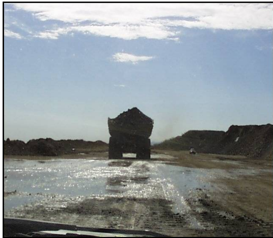
Excess water sprinkling
