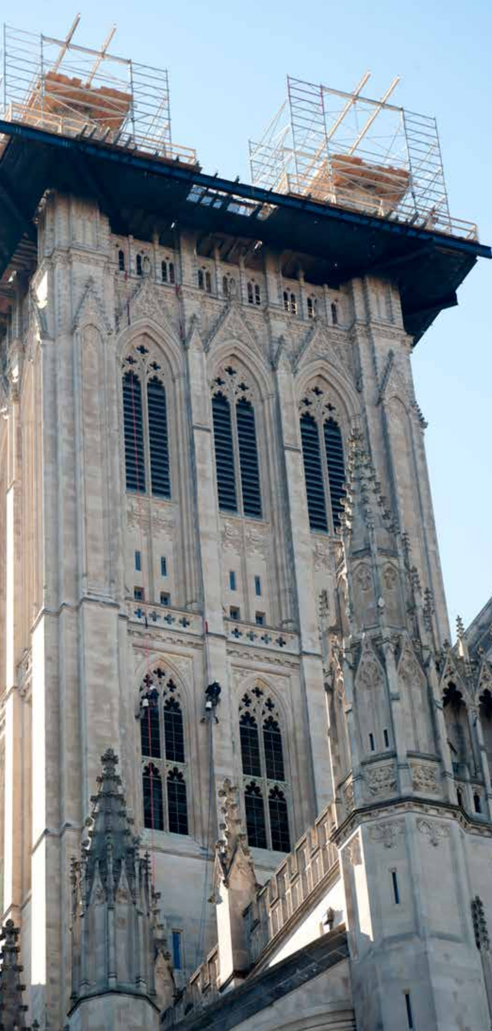
LEFT RAPPELLERS FROM W.J.E. “DIFFICULT ACCESS TEAM” INSPECT THE CENTRAL TOWER FOR LOOSE STONES AND OTHER DAMAGE, NOVEMBER 8, 2011 PHOTO C. STAPERT
