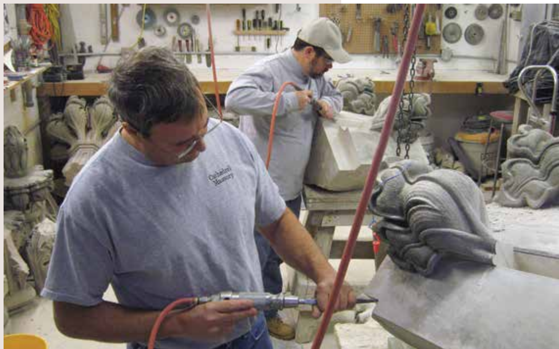
TOP THE TRUCK CARRYING THE PIECES REMOVED FROM THE CENTRAL TOWER GRAND PINNACLES IN FRONT OF THE HERB COTTAGE PHOTO C. STAPERT LEFT CENTER AND BOTTOM DAMAGED CROCKET STONES IN THE CARVING STUDIO RIGHT CENTER ANDY UHL AND SEAN CALLAHAN PREPARING CROCKET STONES FOR "DUTCHMAN PATCHES" PHOTOS J. ALONSO RIGHT BOTTOM JOE ALONSO AND ANDY UHL REMOVE THE DAMAGED GARGOYLE FROM THE SOUTH TRANSEPT PHOTO C. STAPERT
