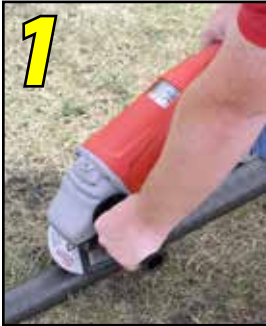
1 Clean pipe before making weld.
