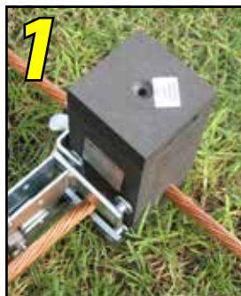
1 Position cleaned conductors in mold.
