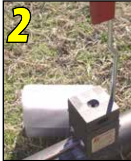
2 Position conductor and mold onto pipe.
