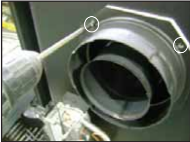
Figure 8.8 Install vent pipe adapter with gasket or high-temp sealant to rear vent opening. Attach with screws removed in Figure 8.5.
