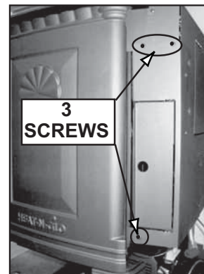
Figure 8.26 Remove valve access cover from back of appliance by removing the three screws indicated.
