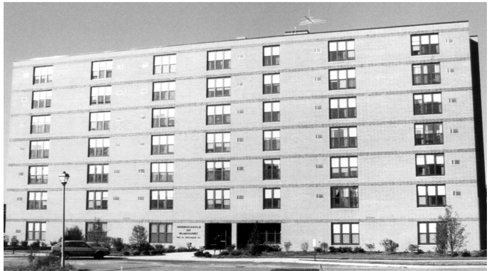
FIG. 3 Green Castle (Elmhurst, IL) is constructed of cavity type bearing walls and spans 7 stories high
