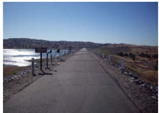
Hidden Dam, Madera County, California: This photo taken on the dam crest at the northwest right abutment looking towards the left abutment.
