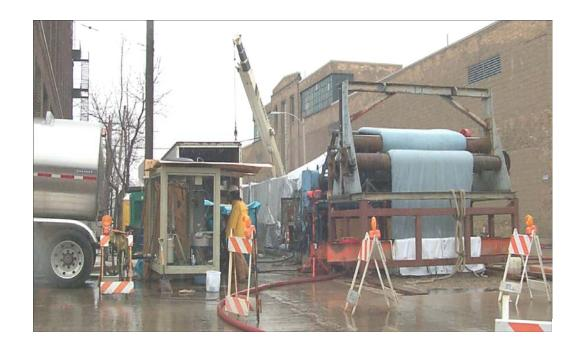
The student learns about the process of impregnating the resin material into the dry tube in a field environment while at the same time installing the liner into the existing pipe.
