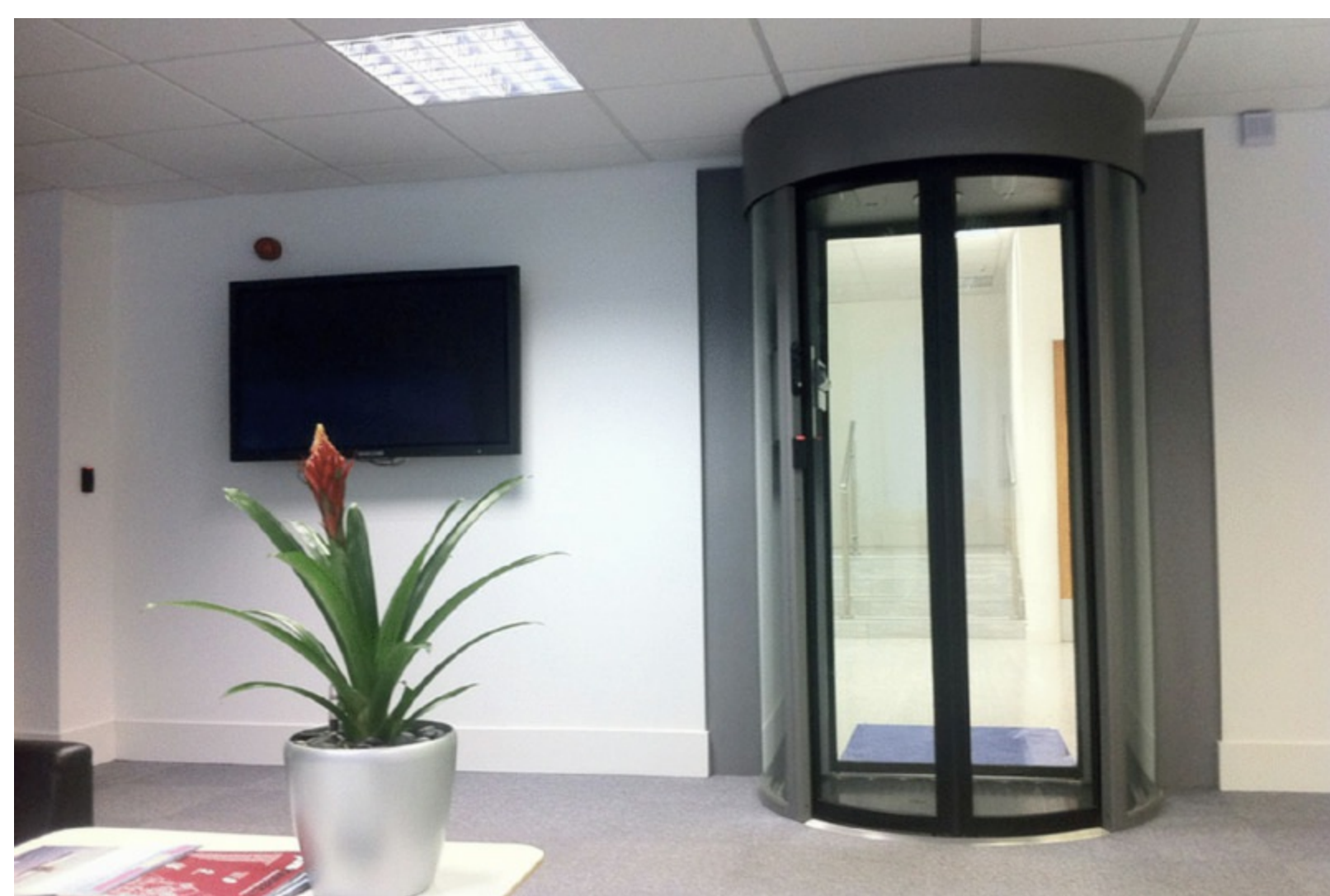
Figure 19.2 A mantrap installed in a lobby
