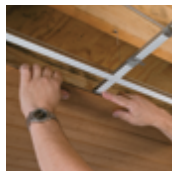
Position planks; slide and secure clips
