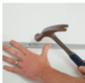
1 Install wall molding
