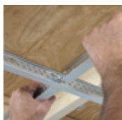
3 Install cross tees
