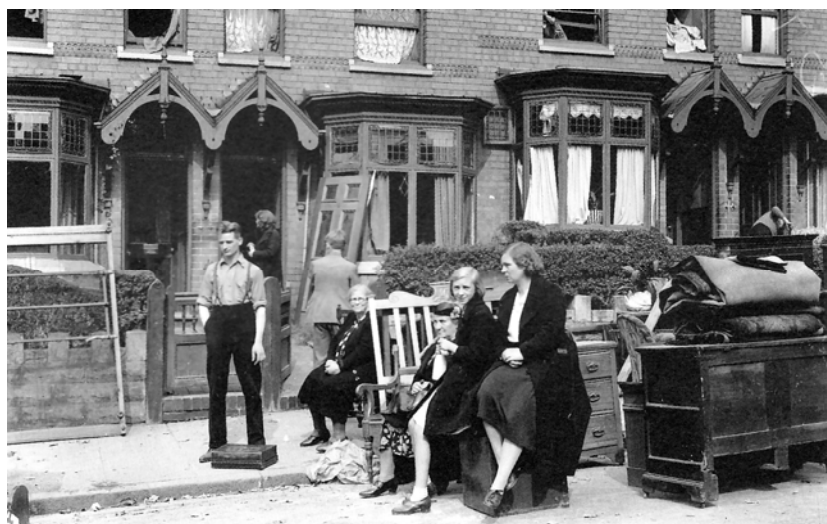
Bomb damage, Stirchley, 1940
