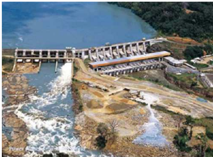
Figure 1: photography of the dam (source: Cameroon-infor.net)
