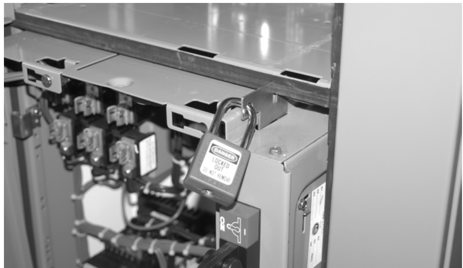
Figure 37 - Unit Interlock to Prevent Insertion - Vertical Operating Handler
