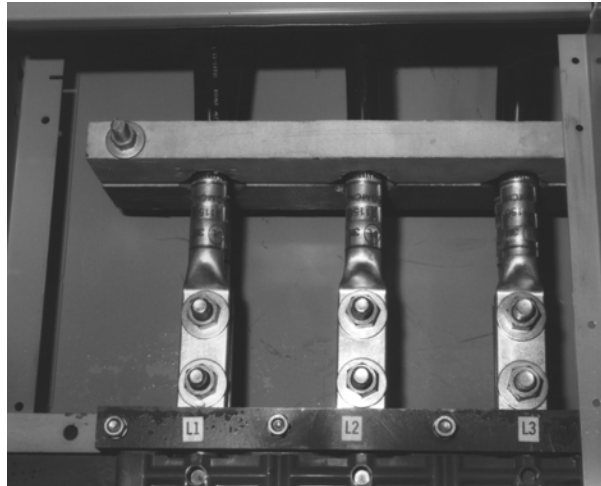
Figure 26 - Securing Cables with Hardwood
