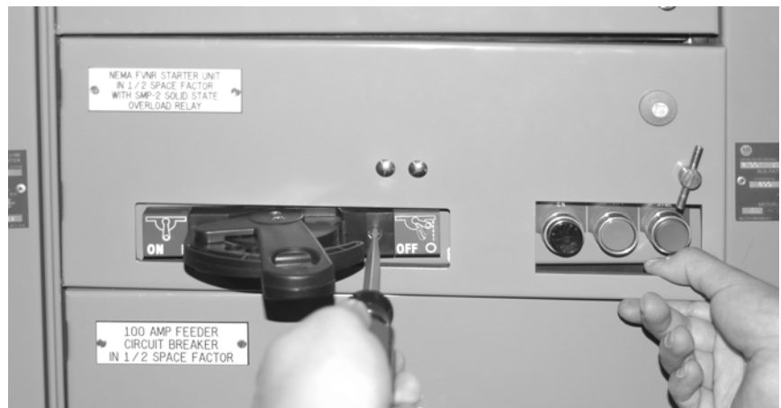
Figure 28 - Operating Handle Defeater for Horizontal Operator Handle
