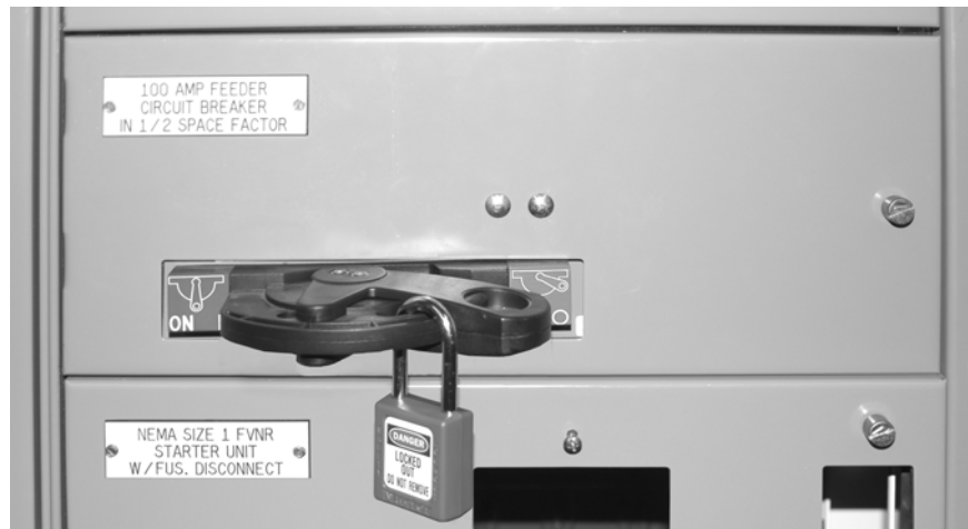
Figure 32 - Locking a Horizontally Mounted Operating Handle in OFF/O Position
