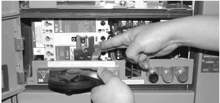
Figure 30 - Defeater Lever for Horizontal Operating Handle
