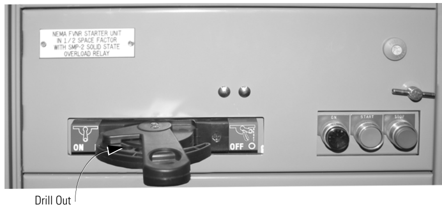
Figure 36 - Locking Horizontal Handle in ON/I Position
