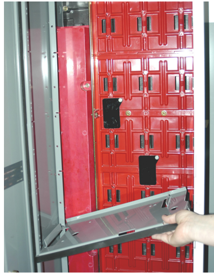
Figure 6 Removal of Support Pan
