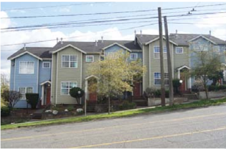
Ground related entrances with residential scaled detailing.
