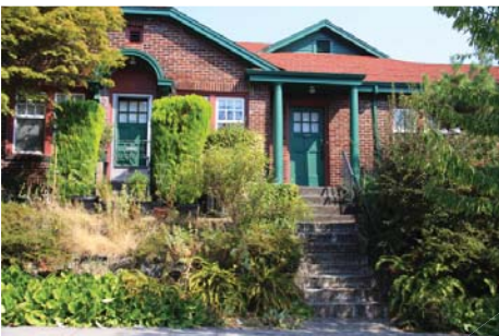
Smaller, single-family scaled bungalow housing with character defining front porch and detailing.
