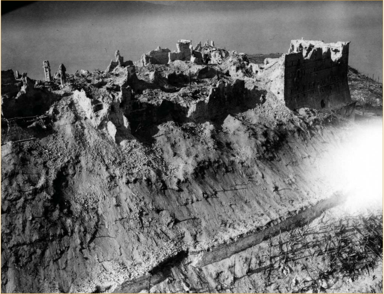
Complete destruction of the Monastery, May 1944
