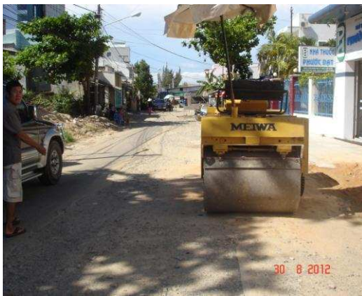
The construction of package BT3/B/10/ICB in Nguyen Hoi Road
