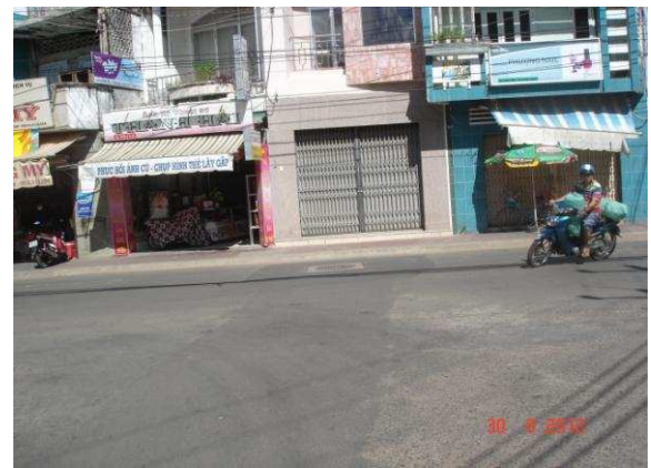
Tran Hung Dao road completed the site in package BT3/B/10/ICB
