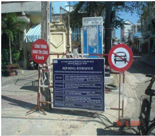
Construction road of package BT5/B/10/NCB
