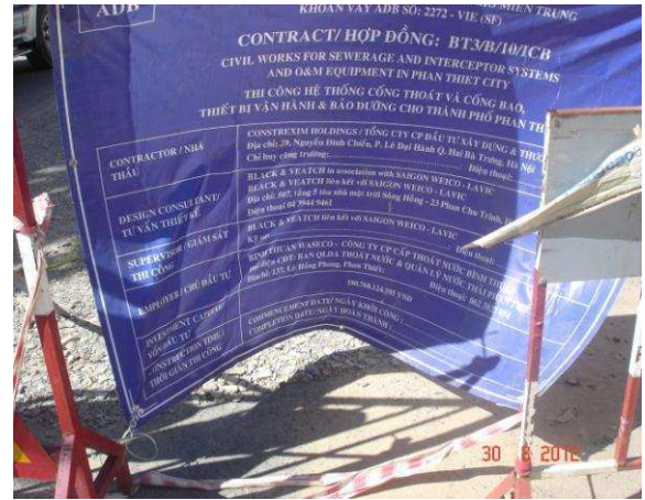
Construction road of package BT3/B/10/ICB
