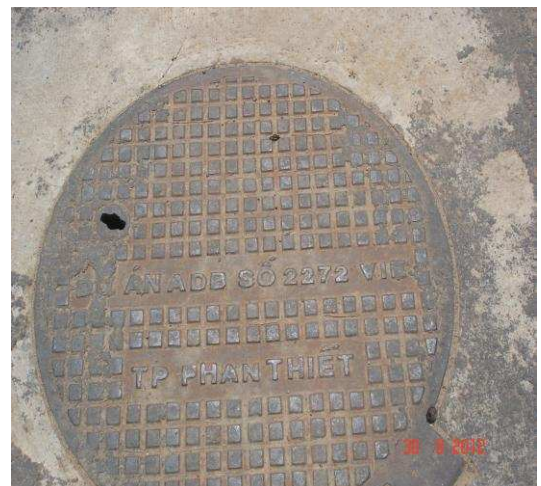
Construction location of Tran Hung Dao Road
