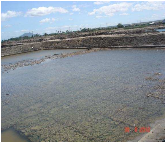
Construction location of wastewater treatment station
