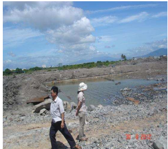
Construction location of wastewater treatment station
