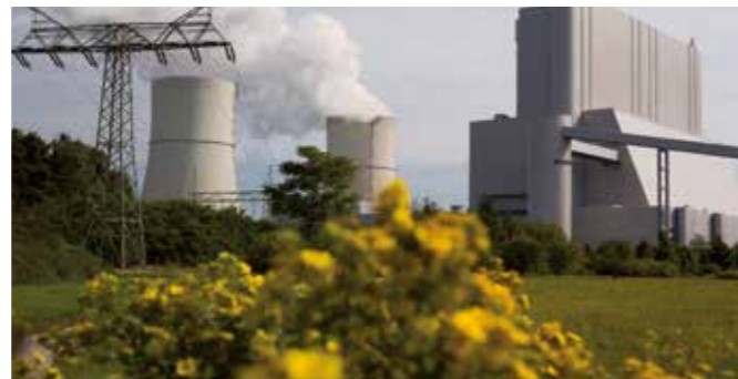
Reliably serving various needs of the power generation industry
