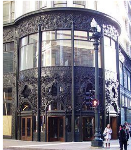
Louis Sullivan, Carson Pirie Scott, 1899–1904, iron, steel, glass, and terra-cotta, Chicago
