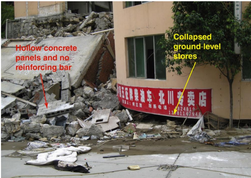
During the 2008 Sichuan, China earthquake, structures of masonry construction, coupled with little or no reinforcing collapsed, leading to tremendous damage and loss of life.
