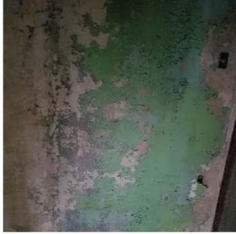
D.) GREEN WALL PRESERVED IN THE HISTORIC JANE ADDAMS HOMES.
