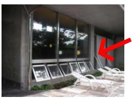
The vertical distance between the inlets and outlets causes the air movement without electricity.
