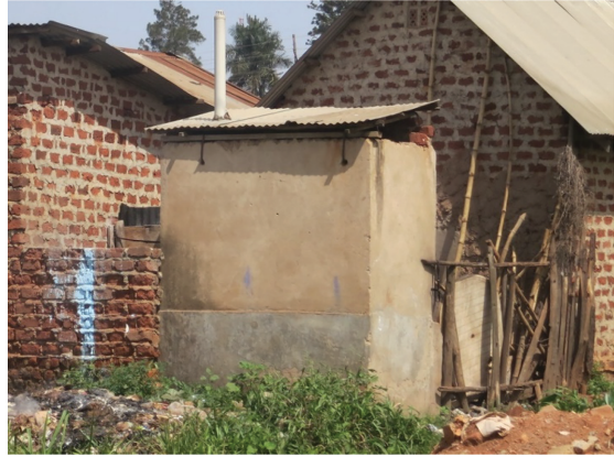
Fig. 6.4 A pit latrine in Kampala, Uganda, an example of onsite sanitation technologies. It stores human excreta in a pit under the toilet and the stored excreta is called faecal sludge (photo credit: Hidenori Harada)
