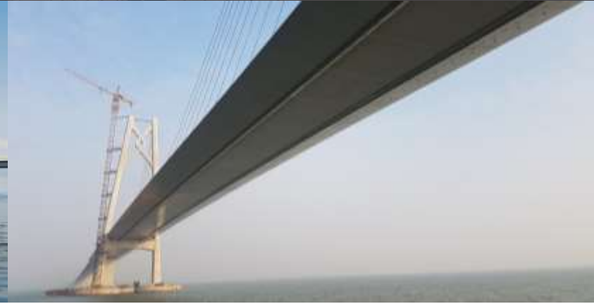
Qinzhou channel bridge
