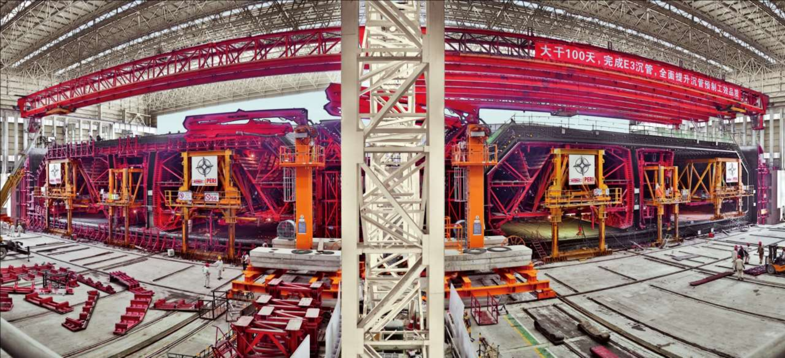
Prefabricated formwork for immersed pipes, designed by Pari, Germany
