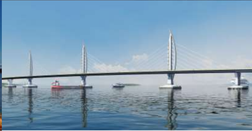
Jianghai channel bridge
