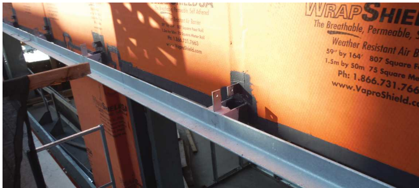
Fig. 1-8 Hot-dipped galvanized standoff shelf angle
