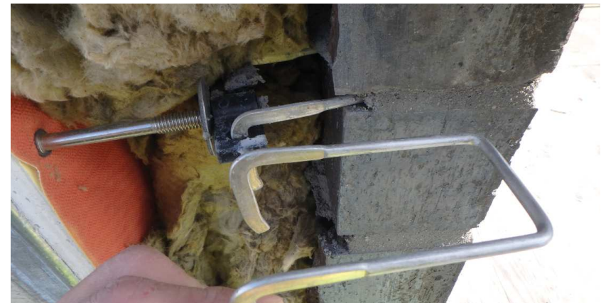
Fig. 1-21 Thermally optimized screw tie with stainless-steel hook and barrel as observed at a freestanding mock-up
