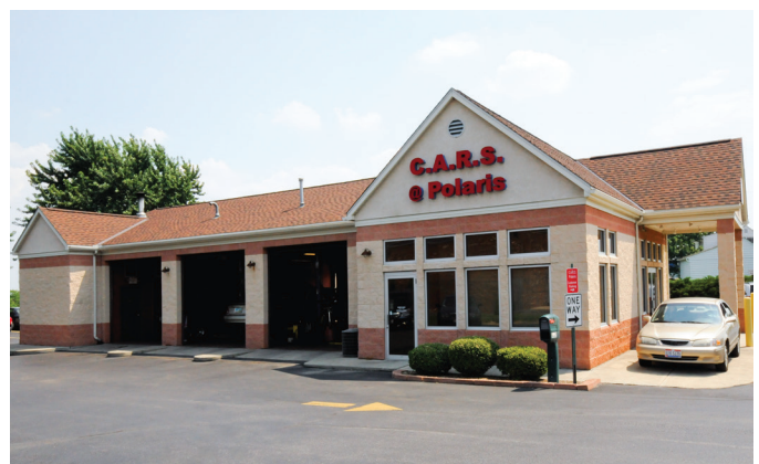
FIGURE 1-4 Automotive repair shop.
