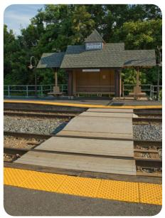
Example of visually contrasting surface materials at a pedestrian crossing. Image: FRA, *Guidance* on Pedestrian Safety at or Near Passenger Stations
