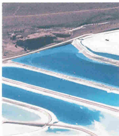
FIGURE 12–10. Brine solutions are evaporated in solar ponds to obtain potassium compounds. The blue dye added to the brine solutions absorbs solar radiation faster and speeds up evaporation.
