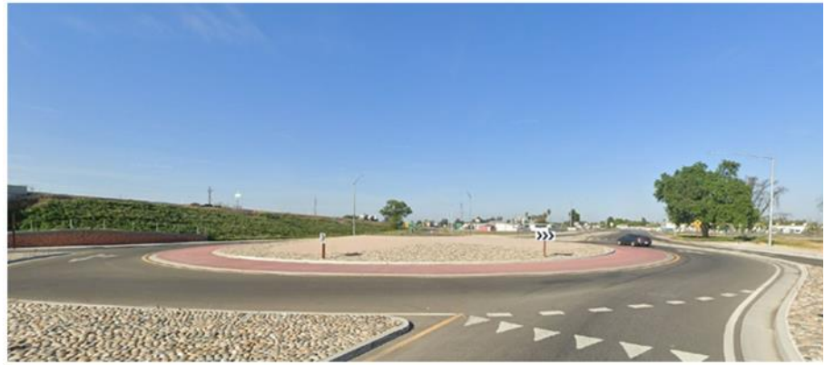
Roundabout that provides range of textures, colors, and shapes to achieve contrast. This example includes a rock blanket on the splitter islands, sidewalk buffer, and a wave pattern on the central island. Contrasting the rock blanket in the central island is tan concrete with brick texturing. Further contrast is provided by the red brushed concrete apron and a small circular landscaped area in the central island. The truck apron is red brushed concrete. The rock blanket could be placed in pervious concrete if needed for stormwater management purposes. Location is Handford Armona Rd at Exit 84 on State Route 198 in Handford, CA.
