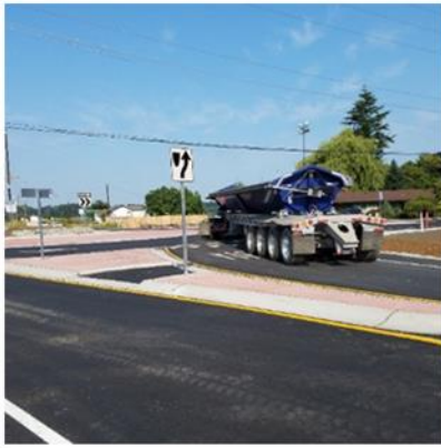
Roundabout showing red concrete with brick texturing for the splitter island and central island, landscaped central island, and gravel and natural plantings at the edge of pavement. Location is State Route 9 at Francis Rd in Skagit County, WA
