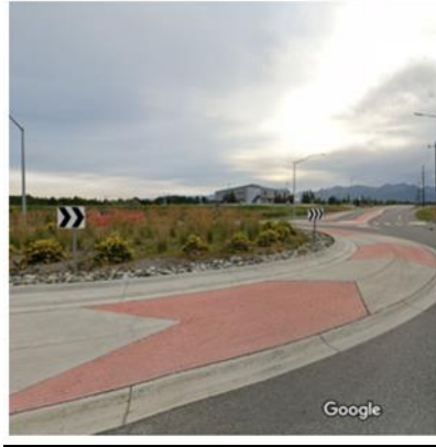
Roundabout apron with a chevron pattern at West 100th Ave and Northbound ramp terminal at the Walter J. Hickel Parkway, Anchorage, AK
