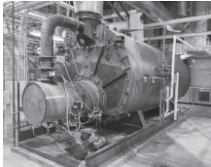
Figure 14.7 Fire tube boilers.
