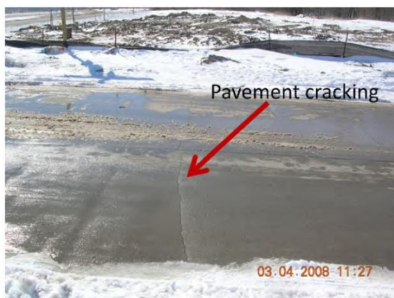
Figure 14B-2.07: Pavement Cracking Caused by HDD Installation
