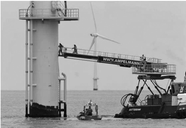
Figure 37: Ampelmann system for accessing offshore wind turbines.
