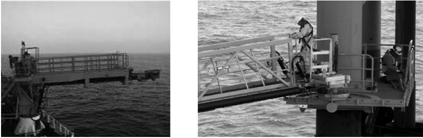
Figure 36: Access to offshore structure with OAS.
