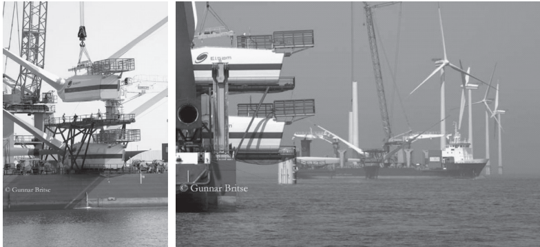
Figure 7: Bunny ears, the pre-fitting of two blades, purpose-converted installation vessels, pre-fitting of J-tube to the transition piece and the installation of the transition piece.
