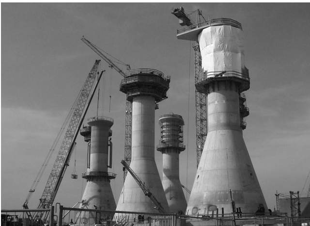
Figure 18: GBSs for Thornton Bank, off the coast of Belgium.
