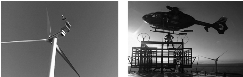
Figure 8: Heli-hoist platforms are installed on turbines to lower mechanics for maintenance.
