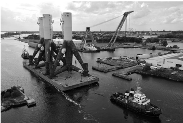
Figure 16: Tripods on a barge, on their way to the Alpha Ventus wind farm.
