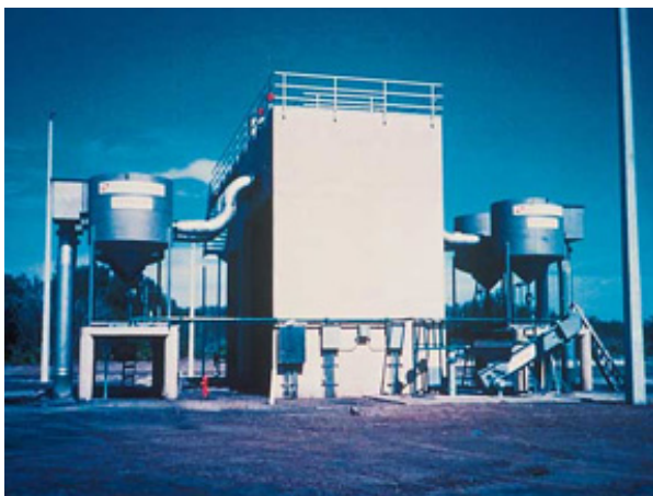
Figure 2.21 “Teacup” Grit Removal Chamber
