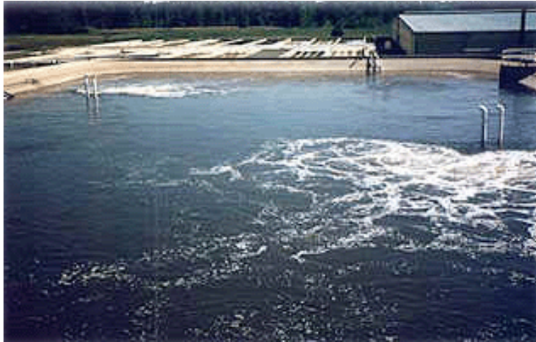
9 10 11 Figure 2.30 Photo of a Flow Equalization System 12
