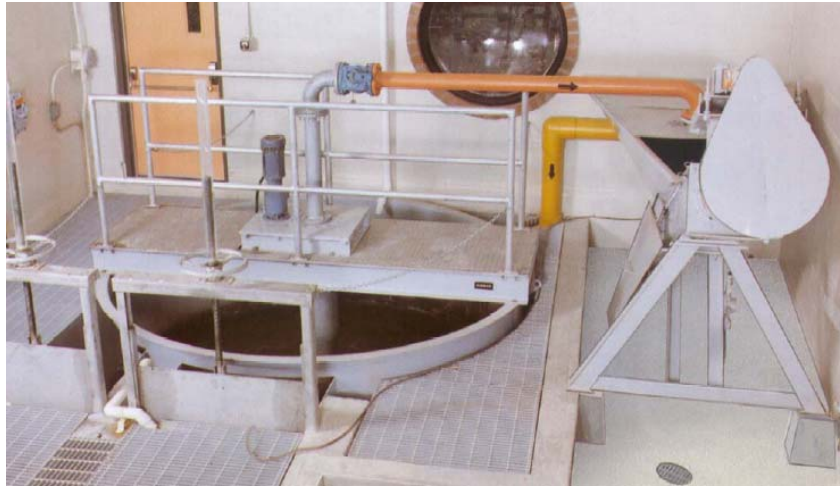
Figure 2.20 Mechanical Vortex Grit Chamber
