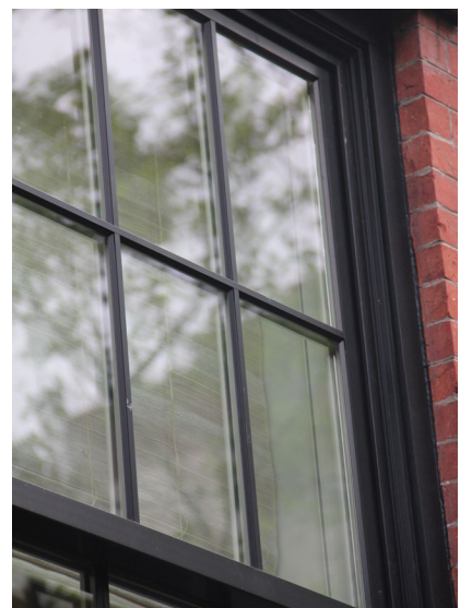
A double-hung replacement window with simulated divided light muntins, featuring exterior and interior muntins, and spacers within the double glazing.
