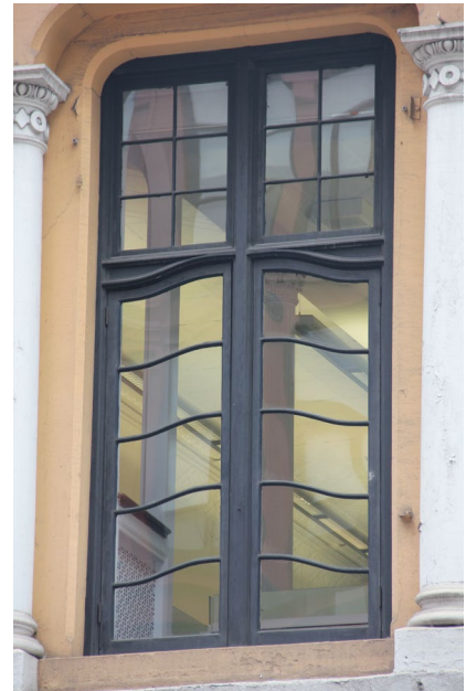
Special window featuring an arched casement sash and curved muntins.
