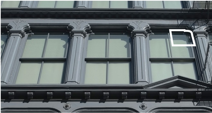
Special window featuring complex corners at the upper sash.
