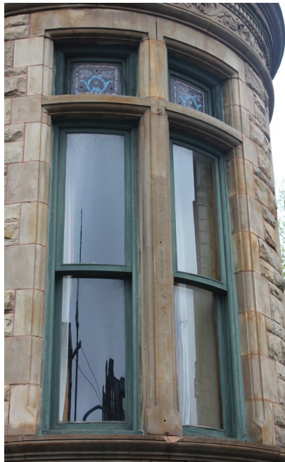
Special window featuring curved sash and glazing, an example of a unique typology.
