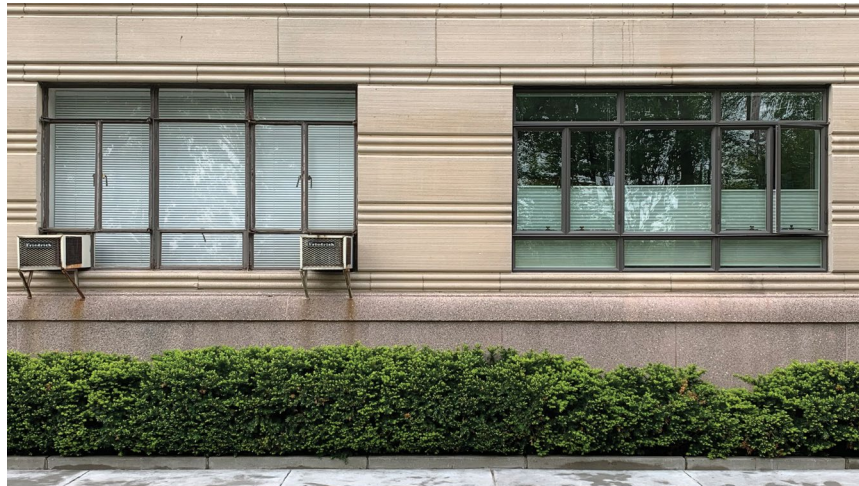
A steel casement window (left) and a fiberglass replacement window (right).
