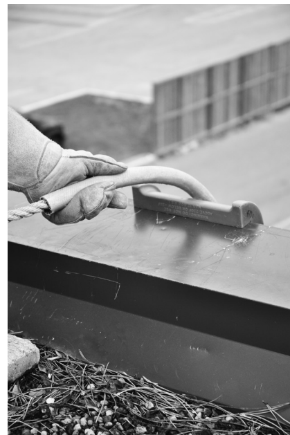
Figure 23-6: Rubber Hose Clamped to Lifeline
