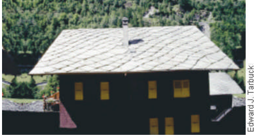
Figure 4 The roof on this house is made of slate. Slate is a metamorphic rock that forms from the sedimentary rock shale. Explaining How can shale become slate?
