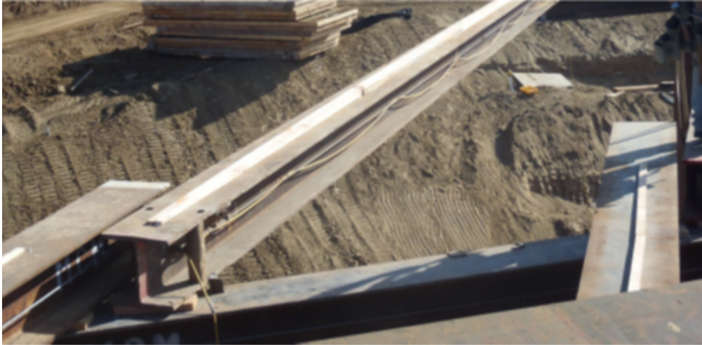
Figure 4-1. Sleeper on the Falsework Stringer
