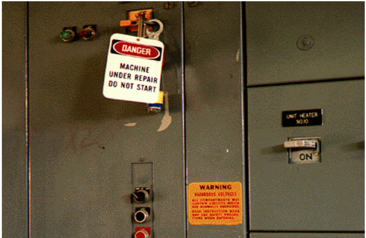
Figure 4.15 Lockout Tagout at Control Panel
