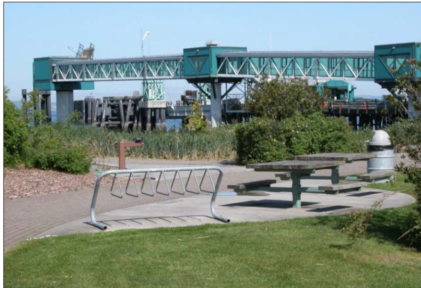
Site Furnishings at Edmonds Ferry Terminal Exhibit 460-8
