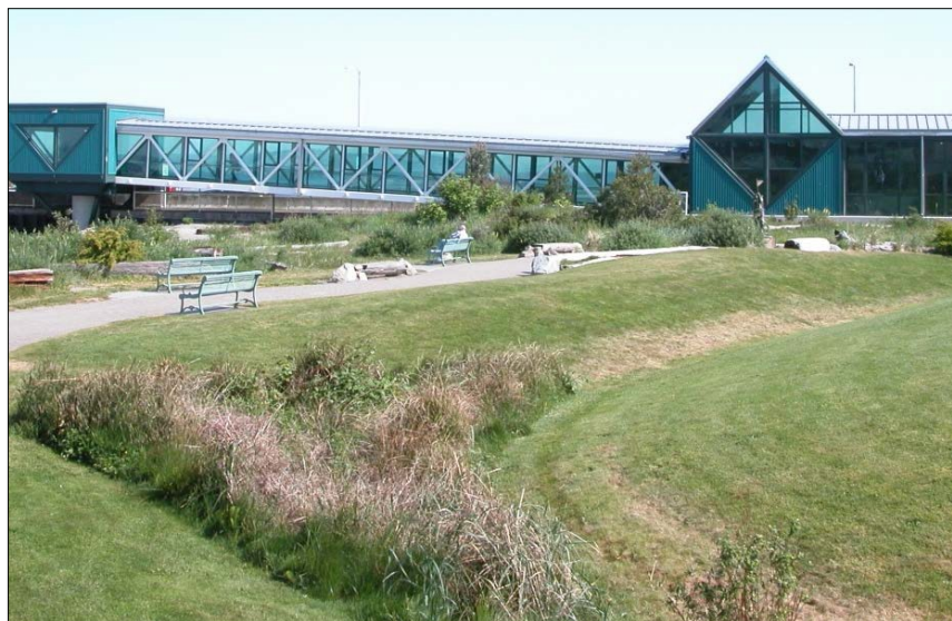
Bioretention Area Near Edmonds Ferry Terminal Exhibit 460-7
