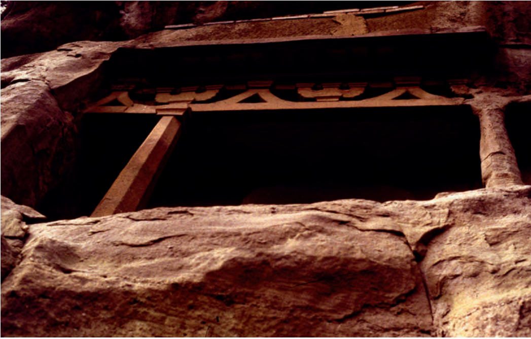
5.24. Entryway showing alternating inverted-V-shaped braces with single-arm bracket sets and red-brown rafters painted under eaves, cave 16, Tianlongshan, sixth century with later repairs
