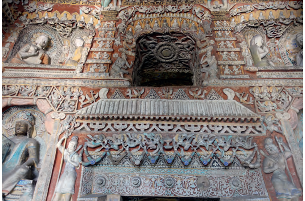
5.19. Detail of Yungang cave 9 showing hip-roofed structure with parallel rafters, under-eave circular rafters with lotus patterns, alternating single-step bracket sets and inverted-V-shaped braces, and segmented arch above Buddha image on either side, 470–493
