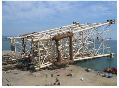
Each topside will be installed with a loadout and installation frame, which can then be moved onto the STB-01 barge. As for the jackets, the barge will be assisted by 3 support vessels during sail-away. Figure 5.13 shows the East Azeri (EA) platform topside on the transportation barge.
