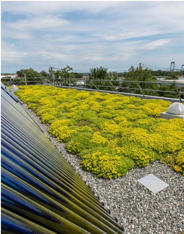
Green Roof at Zerega EMS Station
