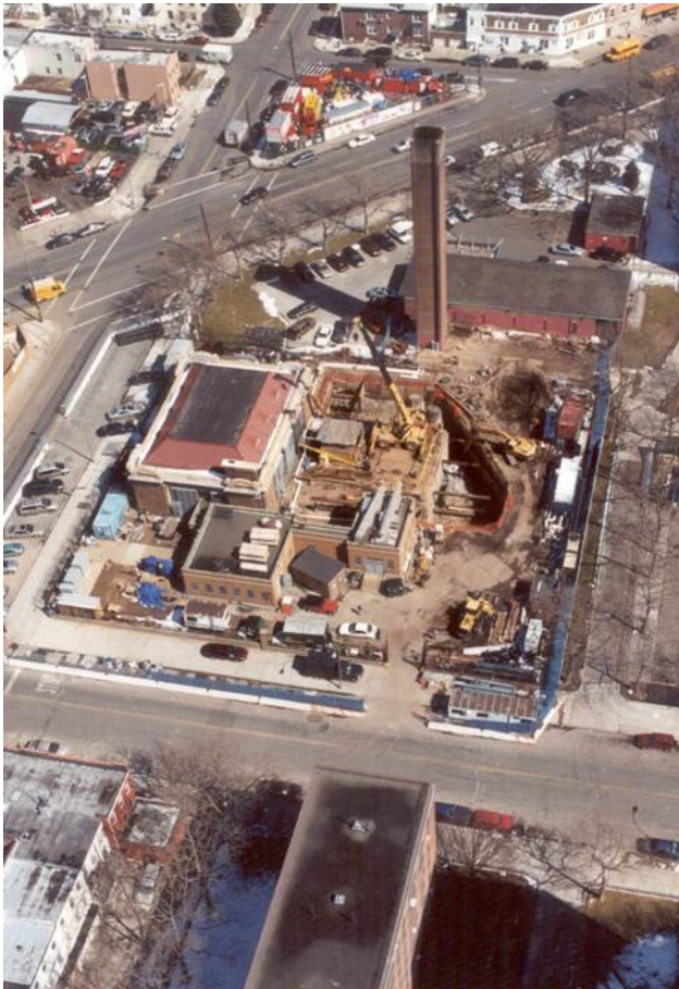
Construction at Avenue V pump station
