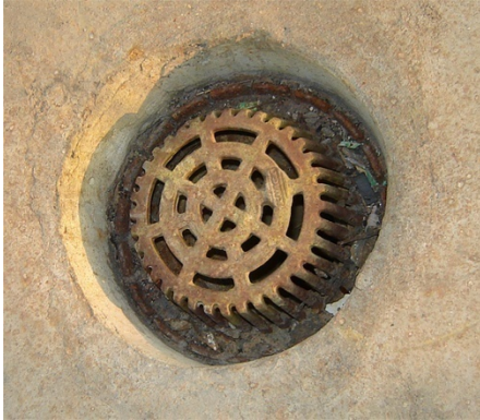
INCORRECT INSTALLATION
