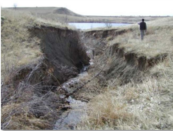
Photograph 8-7. Degraded channel (before restoration).
