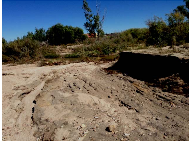
Photograph 8-9. Degradation in a channel.
