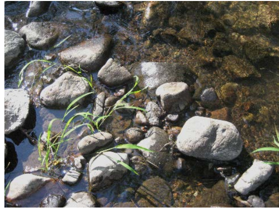
Photograph 8-18. Void-filled riprap is designed to emulate natural riffles, consisting of a mix of rock, gravels and sands that is densely-packed and able to support riparian vegetation.
