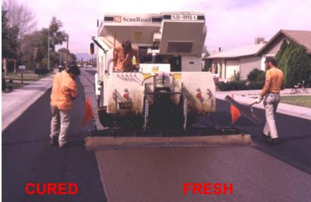
When placed on the pavement surface the mixture breaks and cures creating a new wearing surface.
