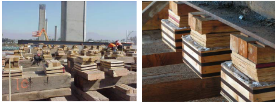
Figure 9-1. Wood Sand Jacks.
