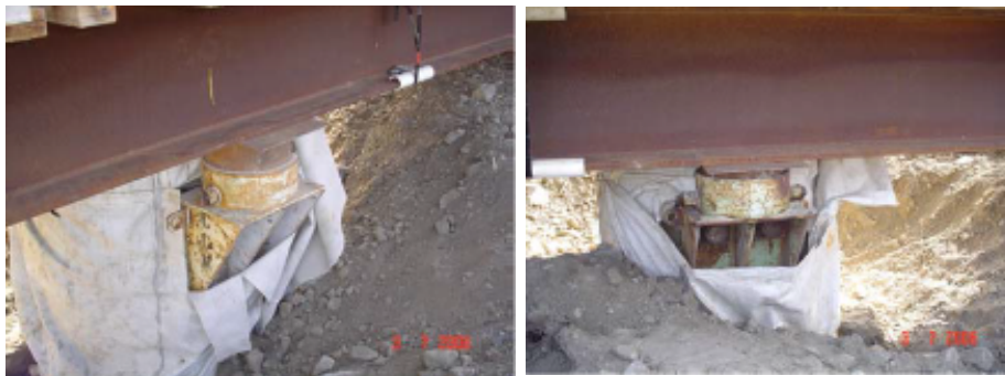
Figure 9-2. Steel Sand Jacks.
