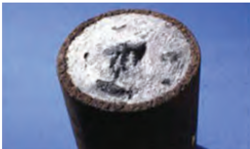
Figure 9.2.8. Boiler tube – scale deposit
