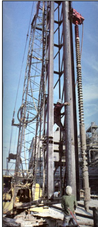
Fig. (9-1) - Creosote-Treated Timber Pile Being Readied for Installation
