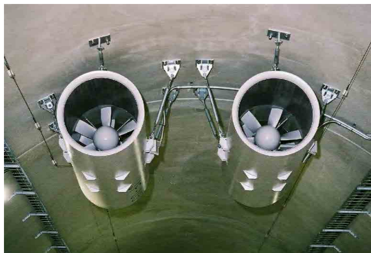
PHOTO 9.9-1 JET FANS INSIDE TUNNEL
