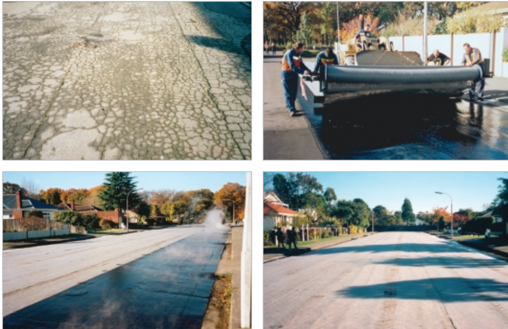
Figure 3-26 Laying a geotextile on a cracked surface.
