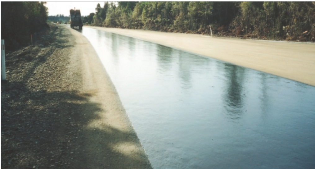
Figure 3-9 A first coat seal under construction on a road on the West Coast of the South Island.
