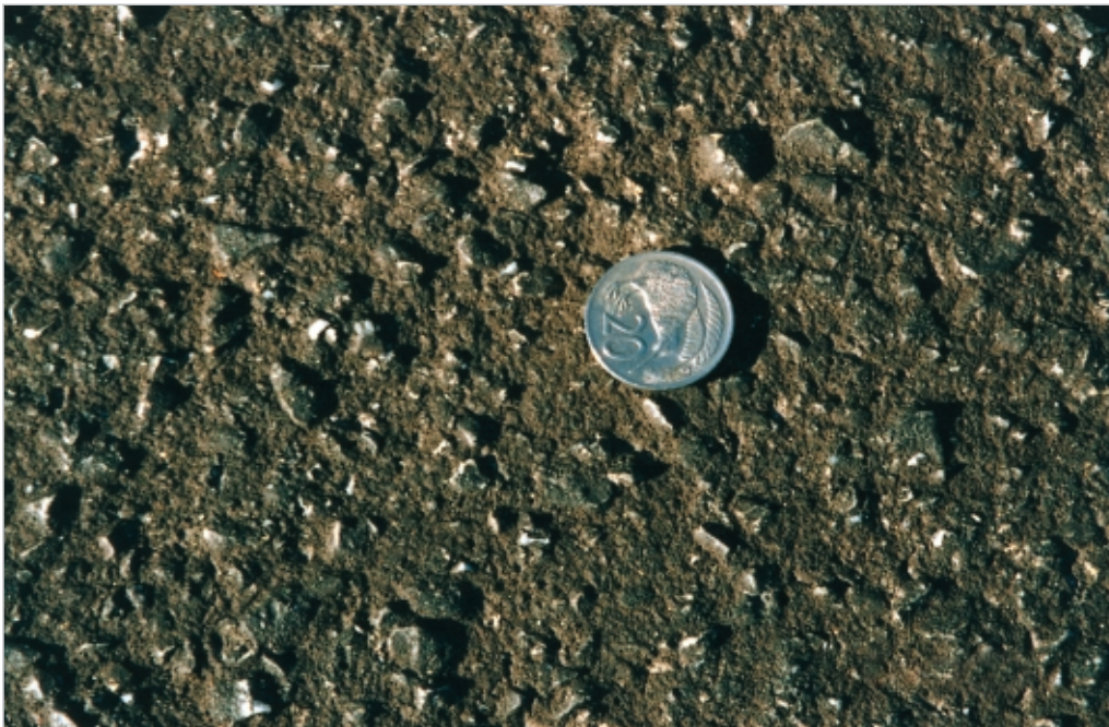
Figure 3-22 Detail of a cape seal surface. (The coin is about 3 cm diameter.)
