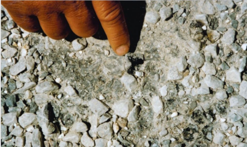
Figure 3-32 Chip loss caused by dirty chip.
